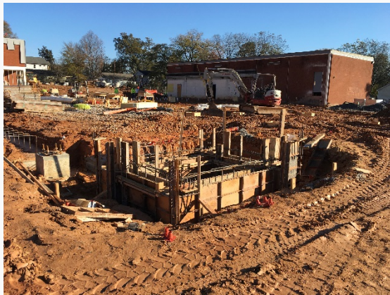
Elevator Pit Formwork
